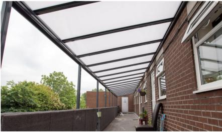
Walkway canopies are purpose built structures designed to provide pedestrians with shelter as they move between buildings, transit stations, parking areas, or other outdoor spaces.
